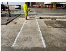
Contingency measures were employed throughout the hangar works, with aircraft rated steel plates, provided to us by BA, available to cover open excavations at the end of each work shift as required.
