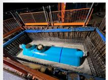
The connection to existing airport drainage systems required excavation of >55m of trench from the proposed location of the new tank installation, with the construction of four access chambers. The drainage trench work and connections to existing airport drainage was completed early in the works program to allow us to hand back the aircraft stand to BA for use as soon as possible.
